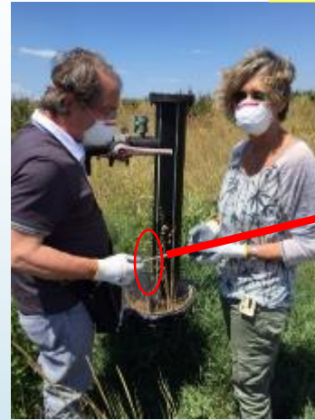
biogas captation tubes
