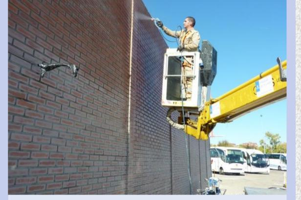
The photocatalytic material (coating) had shown a NO depolluting efficiency of 27% under the ISO international standard [2].
