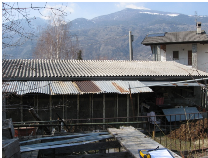
Figure 36. Example of rural roof in asbestos.
