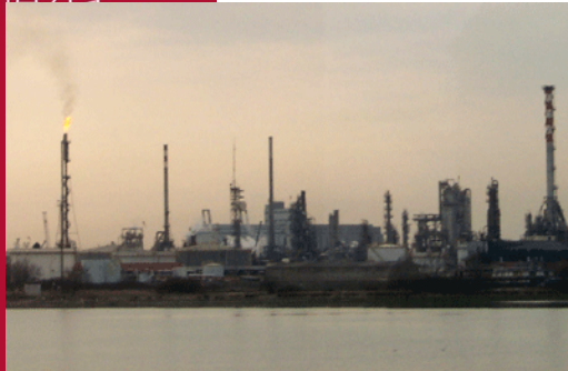
Industrial and energy plants
