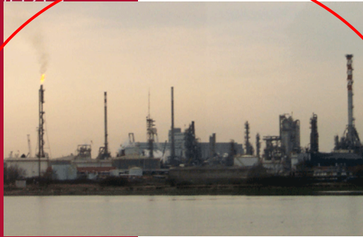
Industrial and energy plants
