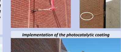
The photocatalytic material (coating) had shown a NO depolluting efficiency of 27% under the ISO international standard [2].
