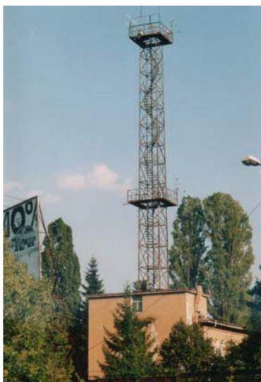
*Figure 1. The meteorological tower with sonic anemometers and a Krypton hygrometer*
