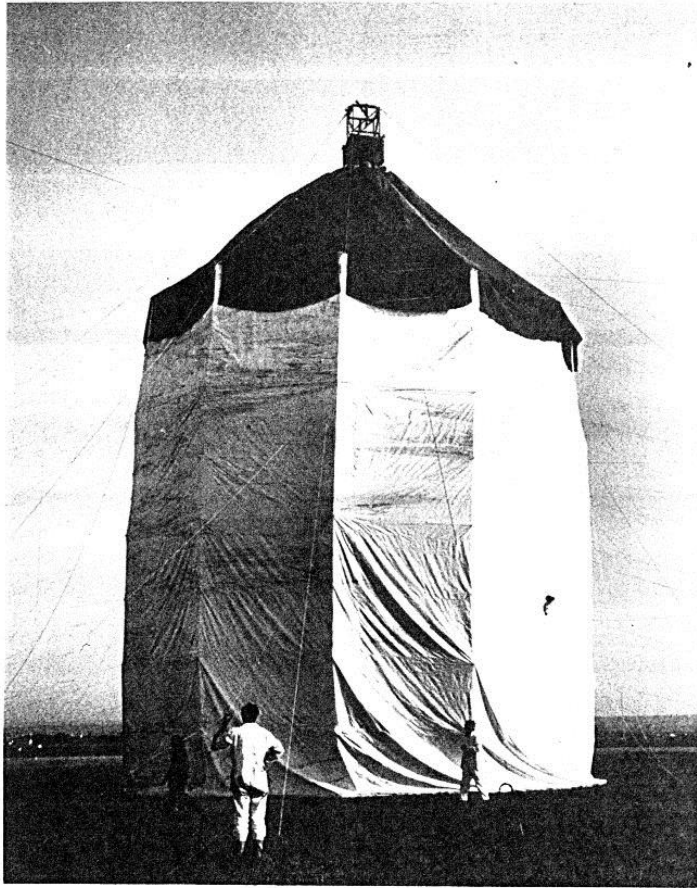
Fig. 8.5 The fully erected gas container
