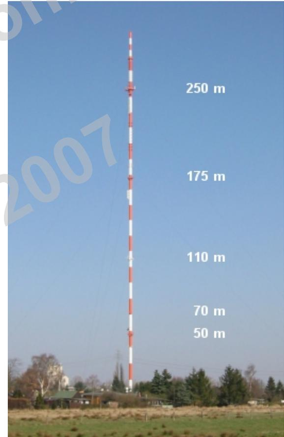
measurements 250 meter tall mast
